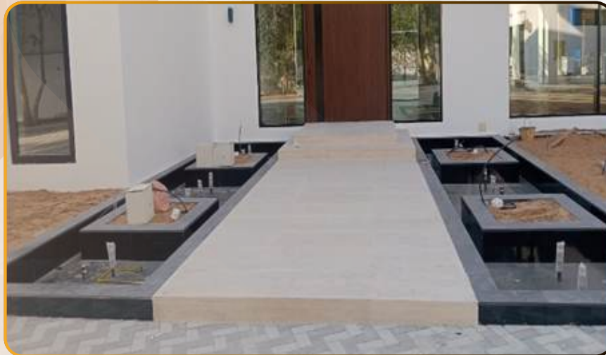
Project: Marbel & Hardscaping Work at Al Barari, Dubai
